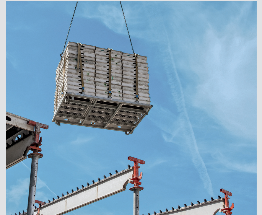
In the large pallets, 48 SKYDECK panels can be stacked and transported very compactly; this corresponds to an area of 54 m 2 .
