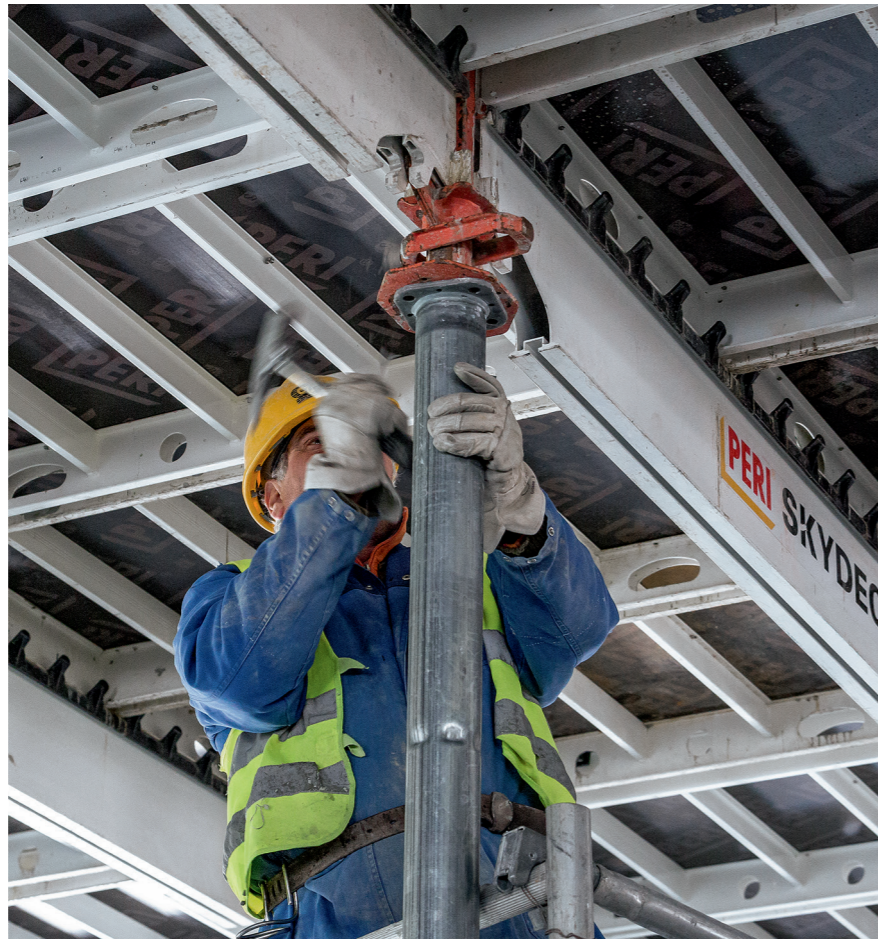
Easy and simple early striking: the formwork is lowered by 6 cm with just one blow of the hammer. After lowering the dropheads, the central panel is removed first followed by the neighbouring panels.
