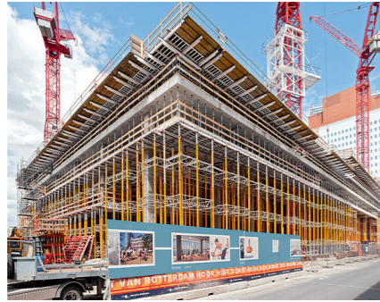
High level of safety at the slab edges
