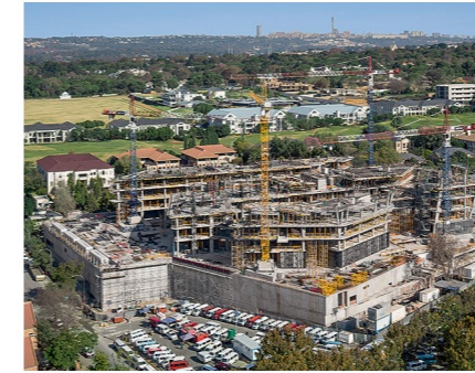
200,000 m 2 floor slabs brought into shape
