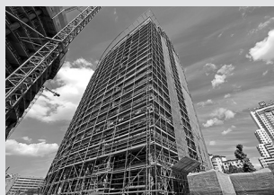
Working scaffolds for facades
