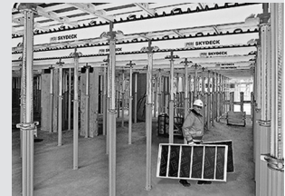
Slab formwork
