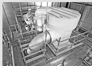
Working scaffolds industry
