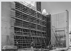
Working scaffolds for construction
