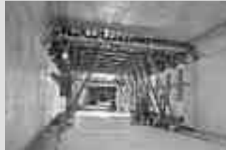
Tunnel Formwork
