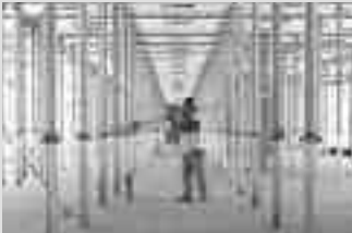
Slab Formwork
