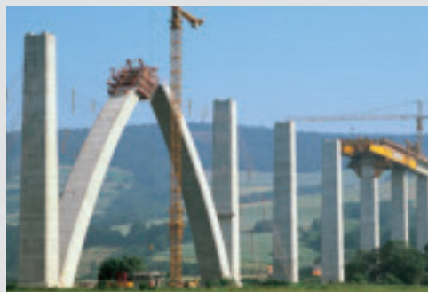
Fuldataal Bridge, Kassel, Germany
