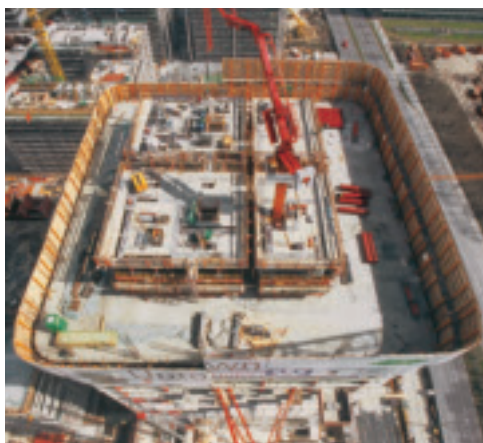
View of the core formwork and climbing protection panel which safely encloses the edges of the building and can be moved by crane.
