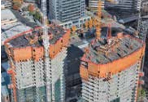
Bellevue Towers, Seattle, USA ACS P and G versions for the core, RCS climbing protection panel on the facade.
