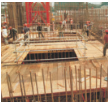
Photo (top): two of the three longitudinal external formwork units have already been raised and are now in position for the next cycle.
