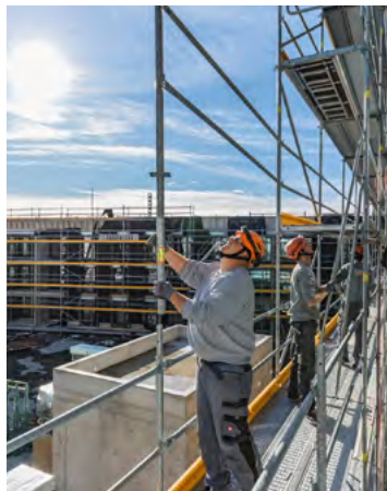
You can attach both guardrail posts to the vertical as well as to the frame and fit or remove them from the level below.
