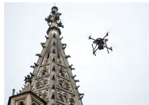
During the renovation of the north-east choir tower, a drone was used for surveying.
