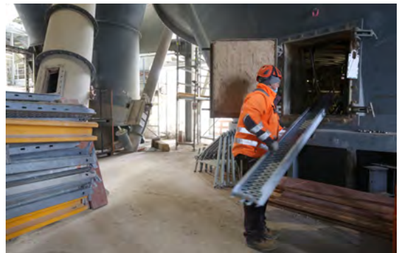
The lightweight, easy-to-handle PERI UP components were fed easily into the facility through small openings and then brought into position.
