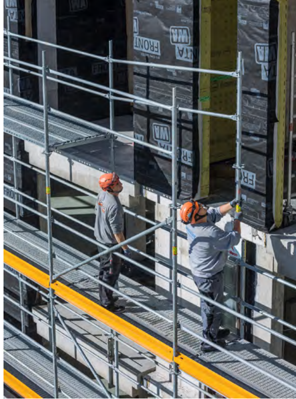
Integrated safety and the guardrail in advance.
