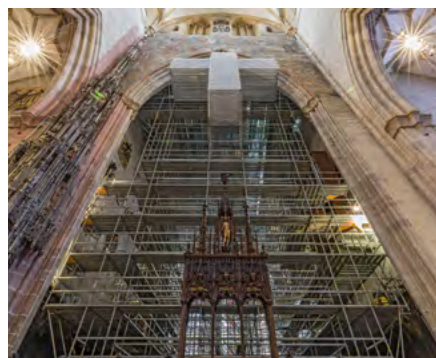
The 13,000 m 3 PERI UP birdcage scaffold in the sanctuary of Ulm Minster was constructed free standing – with no anchoring on the historic building structure.
