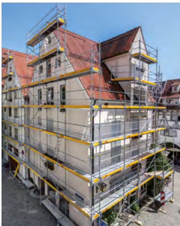
The facade scaffold from the PERI UP Scaffolding Kit is characterised not only by many sophisticated component details but also by the low weight of the individual components. For example, the Easy Standard, weighing only 7.2 kg, makes it easier to transport and erect scaffolding.
