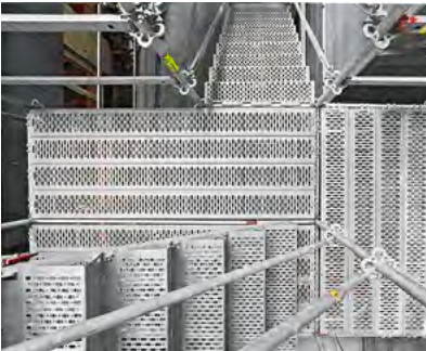
The closed, non-slip decking offers a high level of comfort and safety.
