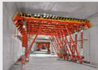
Tunnel Formwork
