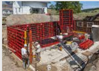
Wall Formwork
