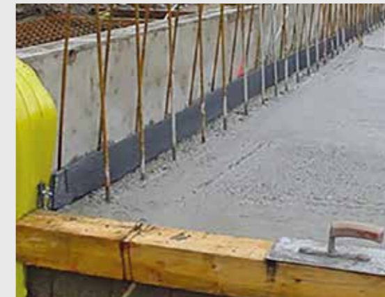
CEMflex Clamping Plate
