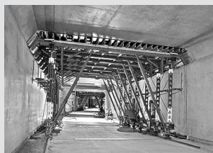
Tunnel Formwork
