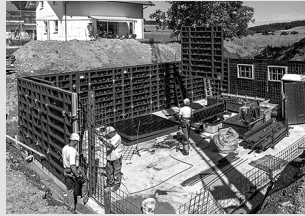
Wall Formwork
