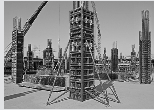
Column Formwork
