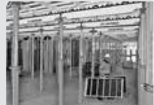
Slab Formwork
